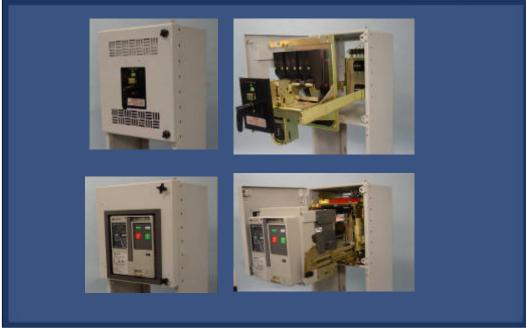
If the breaker switching mechanism itself is in need of replacement, consider installing a form-fitfunction replacement using a modern power circuit breaker in the old draw out mechanism. These new circuit breakers can be mounted into a variety of manufacturer's draw out assemblies. This provides a new warranty and because the breaker is of current design, more easily obtained and less expensive spare parts.
